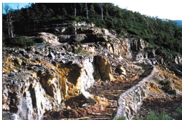
Lune River Quarry rehabilitation with soils spread on benches and cave inflow filters installed, July 1993. Photo by Barry Batchelor – from the Evaluation Report
